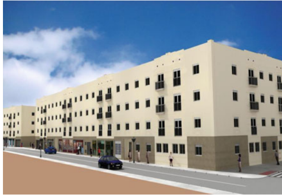
Fig. 1 Type of residential building under analysis
